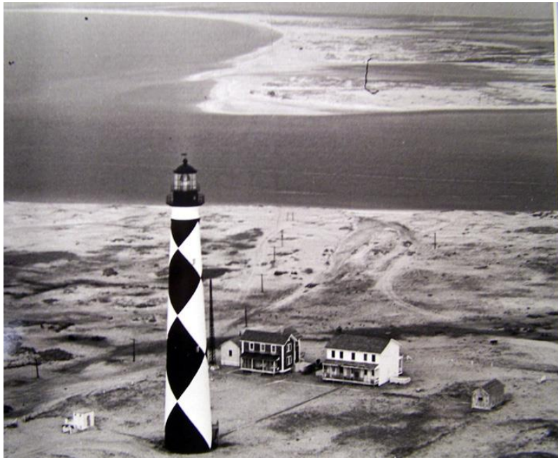
Cape Lookout Light Station c. 1940 Barden Inlet and Shackleford Banks in the background
